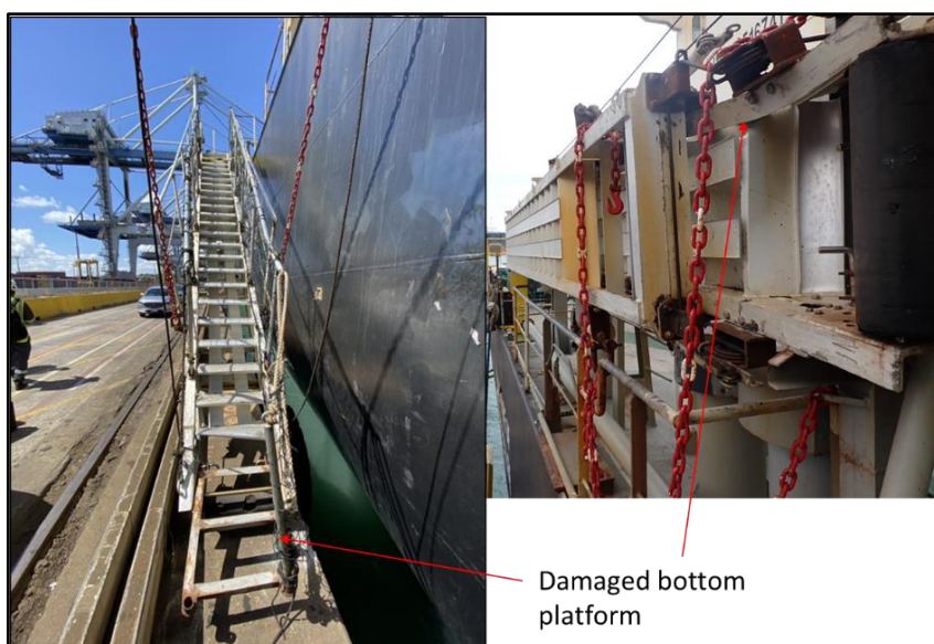
Figure 13: Photos showing damaged bottom platform of accommodation ladder
