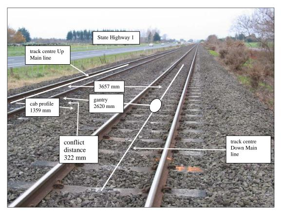
Figure 3 Track, gantry and locomotive clearances at the collision site (not to scale)
