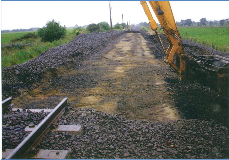
Figure 6 Excavated track formation
