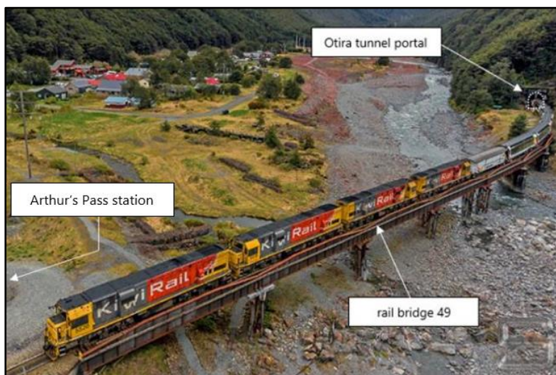
Figure 7: A TranzAlpine exiting the Otira tunnel and crossing bridge 49 at Arthur's Pass (not the train that was involved in the incident)
