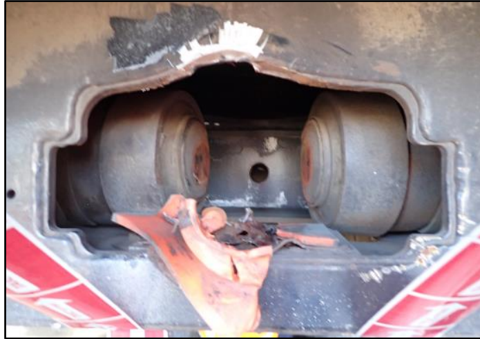
Figure 9: Rear of carriage one showing coupler drawgear location and damaged chassis
