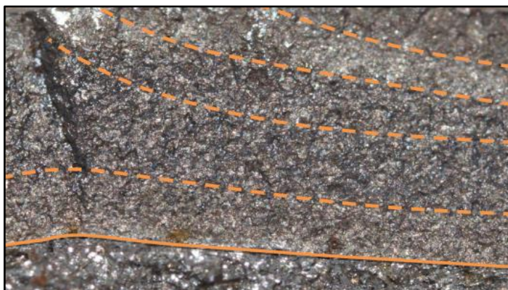
Figure 21: Fatigue crack changes over a period of time
