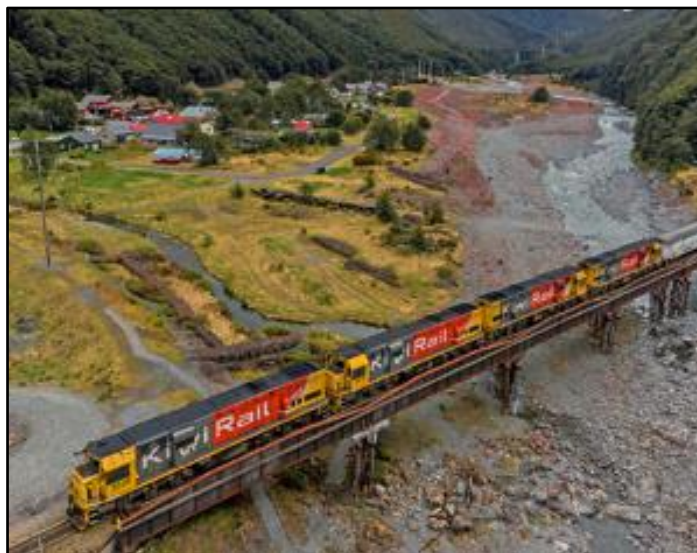
Figure 16: Four locomotives attached to the TranzAlpine
