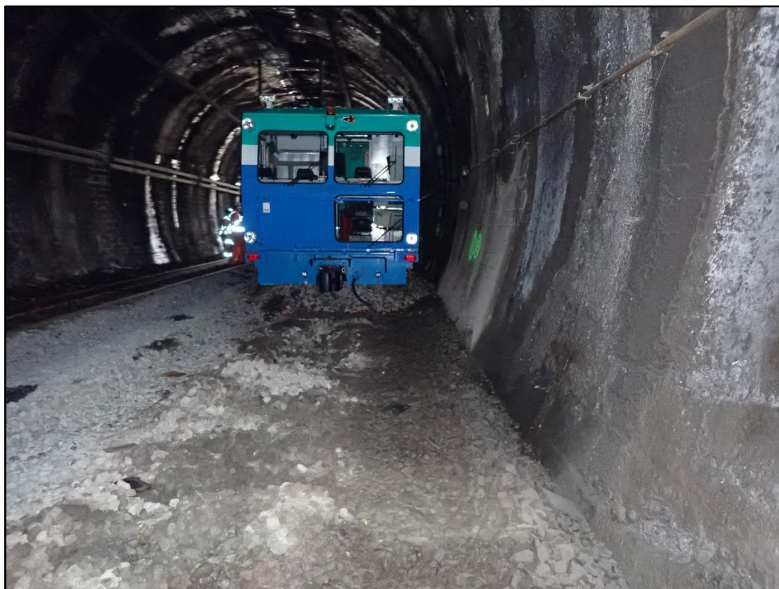
Figure 10: Track removed from tunnel 19 up main line
