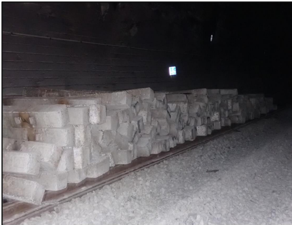
Figure 9: Concrete sleepers stacked on tunnel 19 up main line
