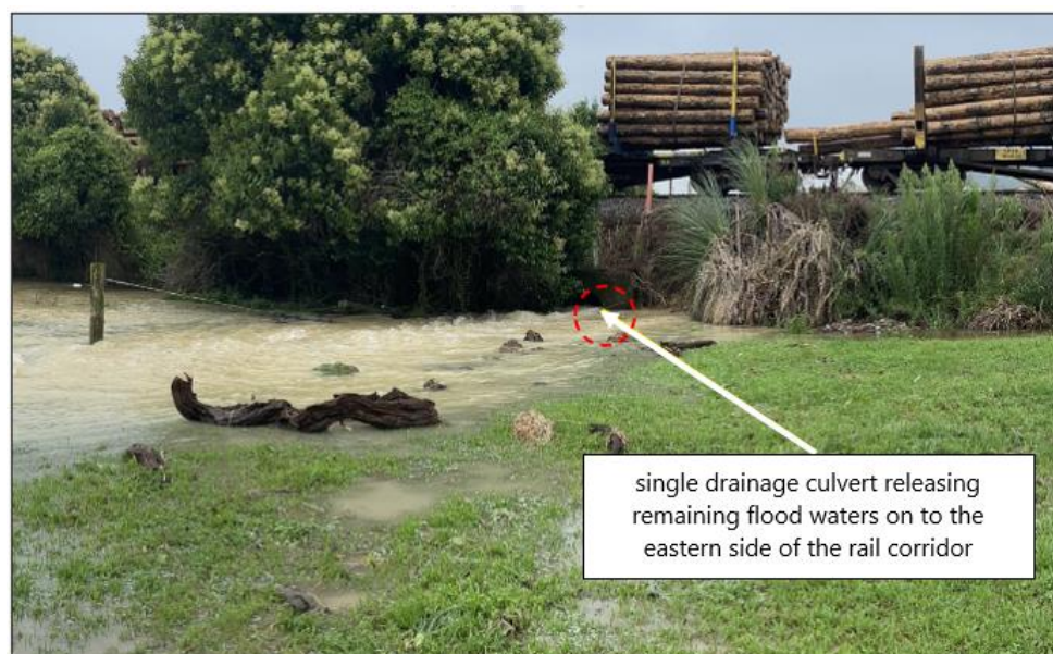
Figure 22: Culvert allowing floodwater to move east onto farmland (Credit: KiwiRail – photograph taken at approximately 10:00 on 29 January)
