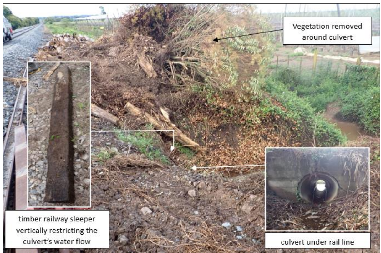
Figure 23: Western entrance of culvert
