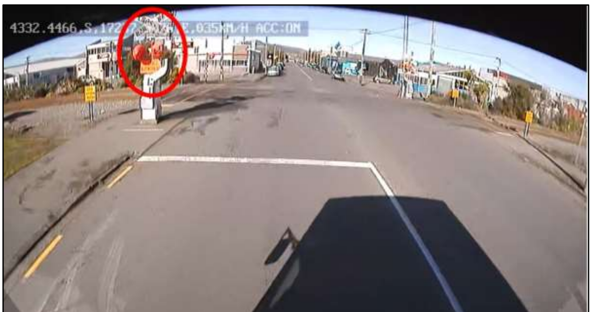
Figure 6: Bus driver's view approaching level crossing – warning lights bagged
