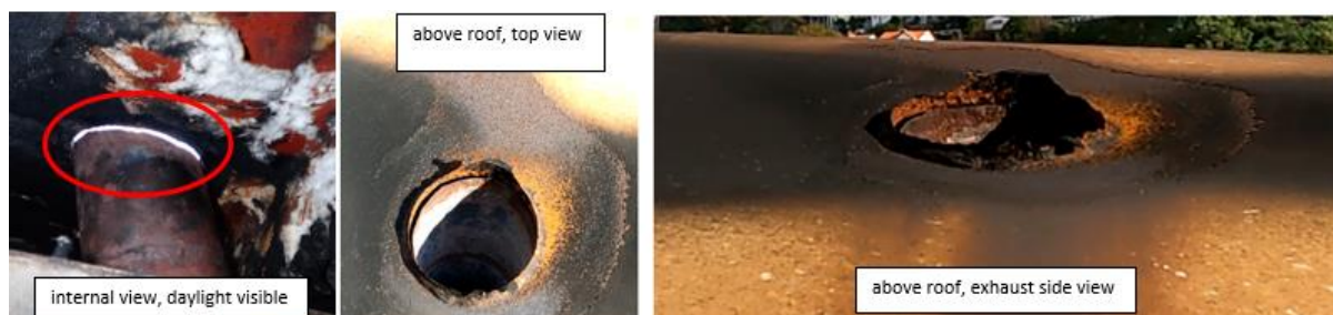
Figure 5: AG130 exhaust tail pipe inside, top and side views
