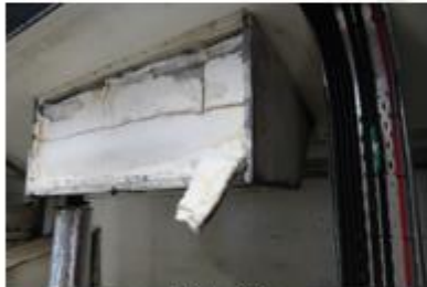
Photo 12. External access cover of exhaust silencer enclosure removed from AG176. IMG_2114.jpg
