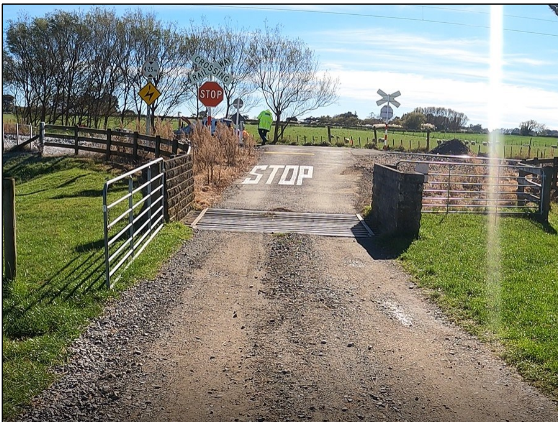
Figure 3: View towards worksite from southern side of crossing
