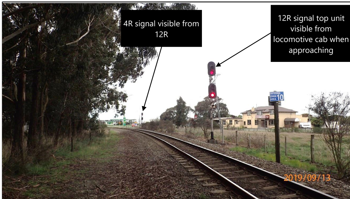
Figure 6: Approach to 12R signal
