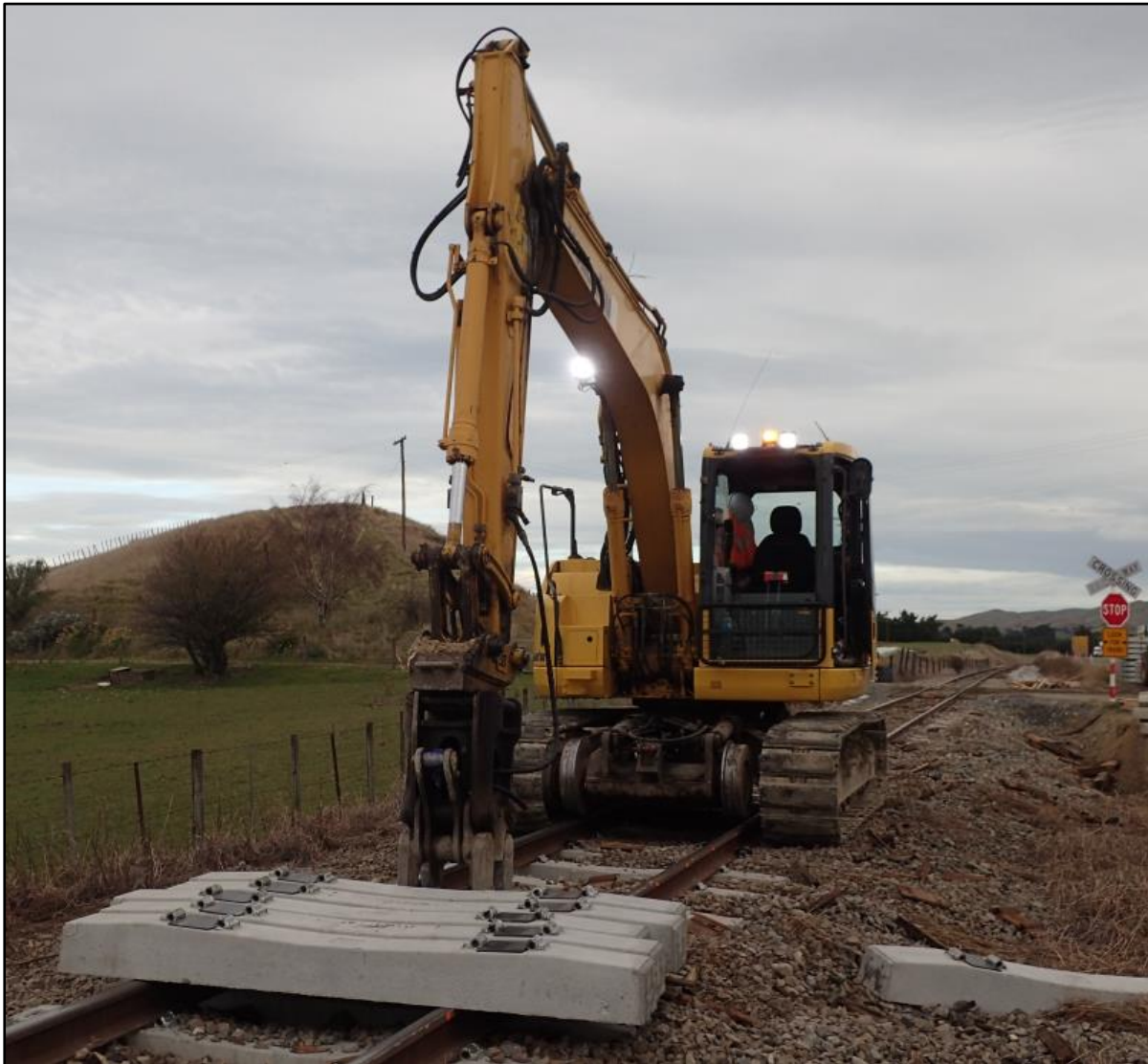
Figure 1: Re-enactment of hi-rail excavator and sleeper position on the track at the location of the incident
