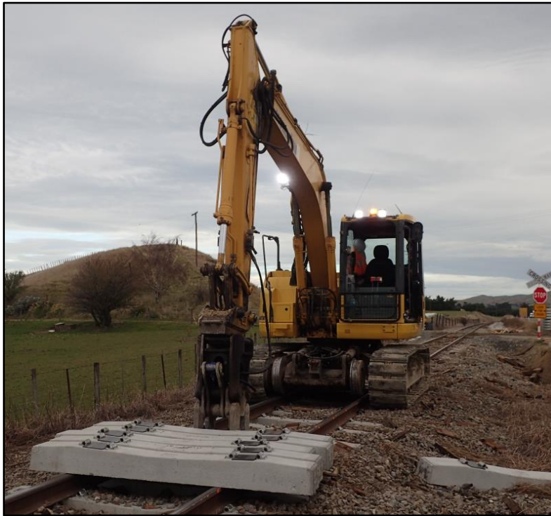
Figure 4: Re-enactment of hi-rail excavator and sleeper position on track
