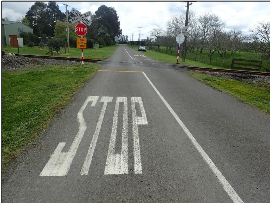
Figure 6 The road markings for the northbound approach to the Lambert Road level crossing
