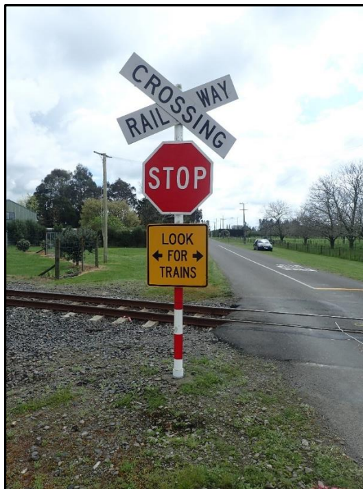
Figure 3 The STOP sign assembly for the northbound approach to the Lambert Road level crossing
