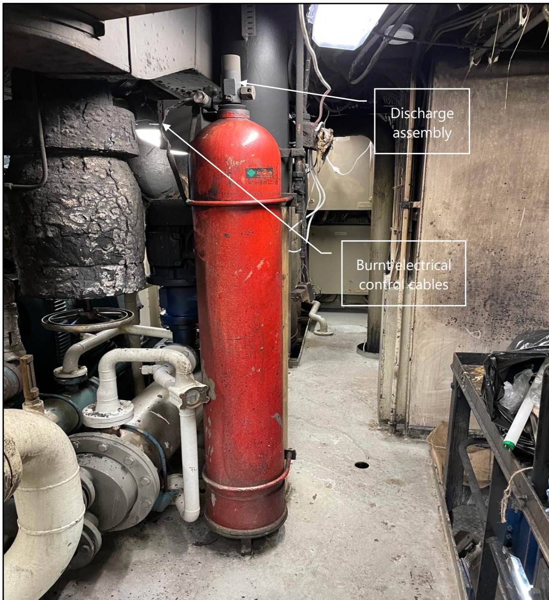
Figure 10: Photograph of Halon bottle near seat of fire
