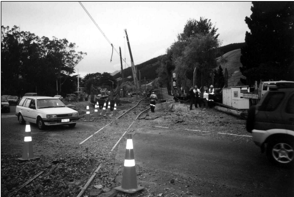
Figure 1 General view of the site
