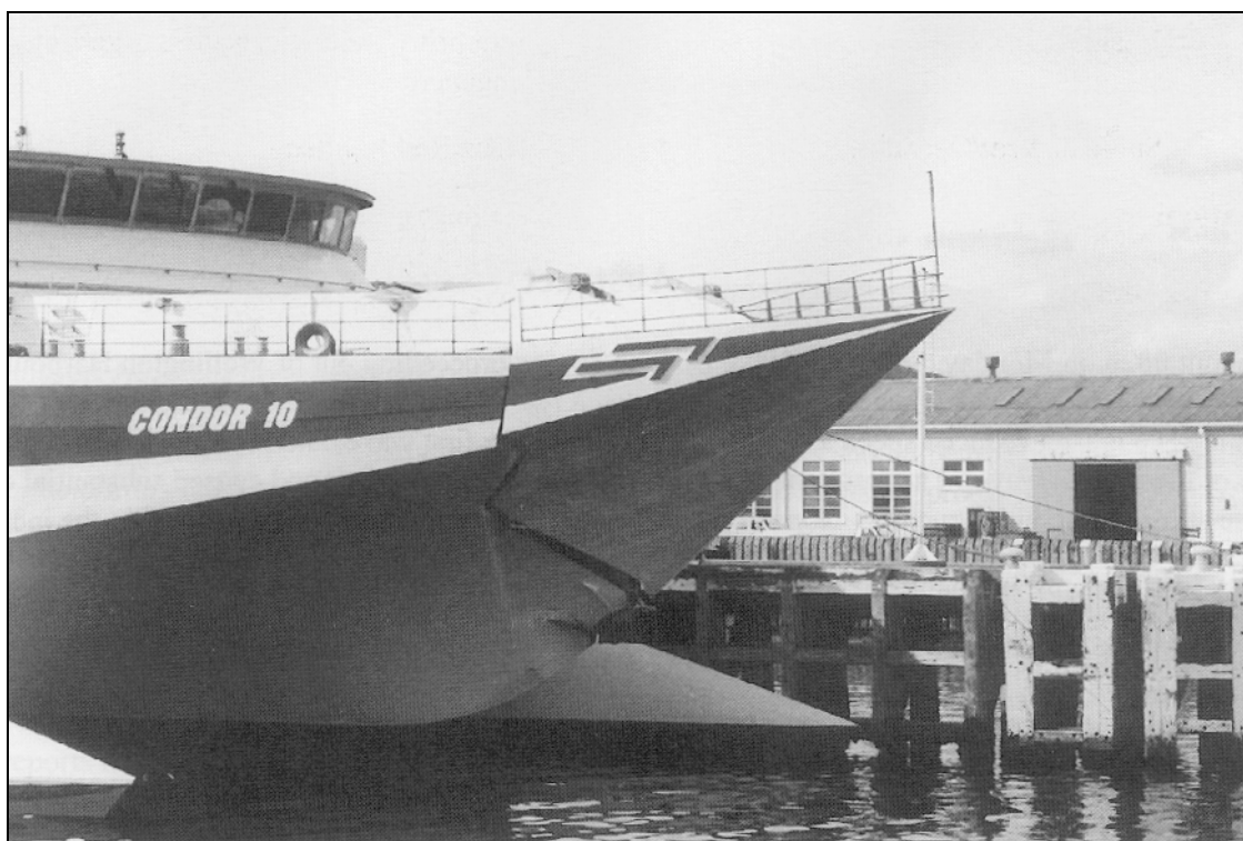
Photograph showing the displaced bow visor on Condor 10 shortly after the incident
