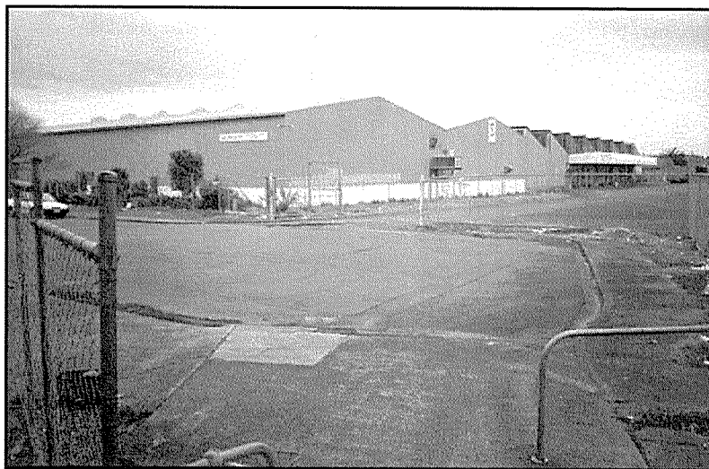
Figure 3 Open gateway entry to the west side of the yard
