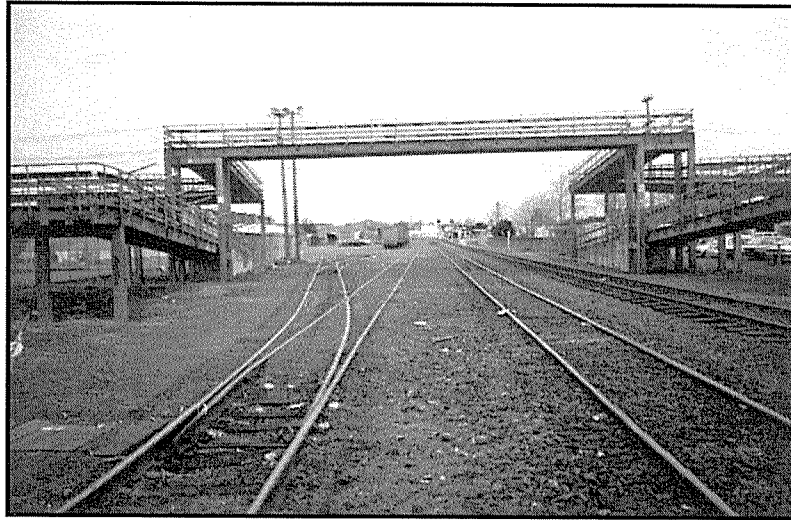
Figure 2 Looking north to the footbridge and crossing point beyond
