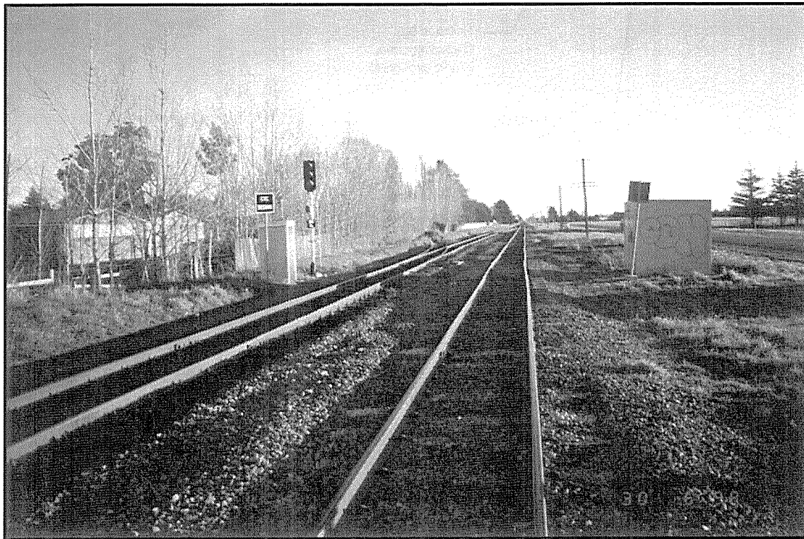
Figure 3 Looking south. Location box on the right containing the crank handle
