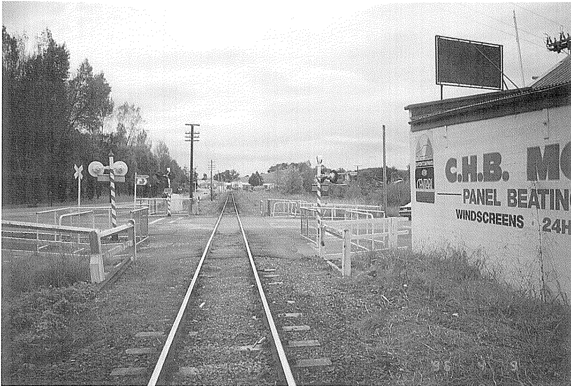
Figure 1 Northbound LE's view of the utilities approach (right hand side)
