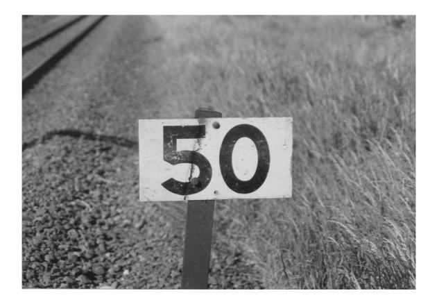
Figure 5 Curve Speed Board following reinstatement
