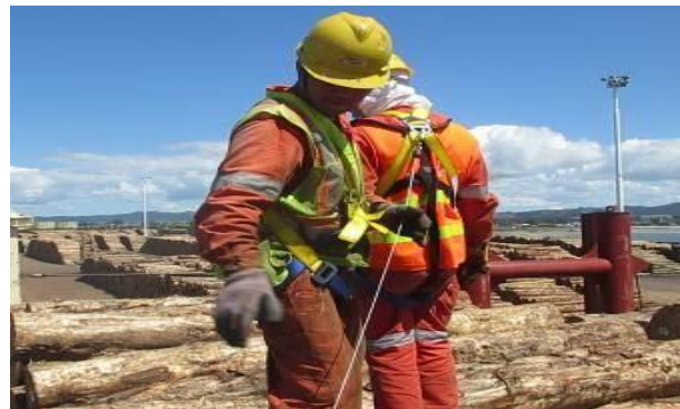
FPD wire end hooked on to safety harness
