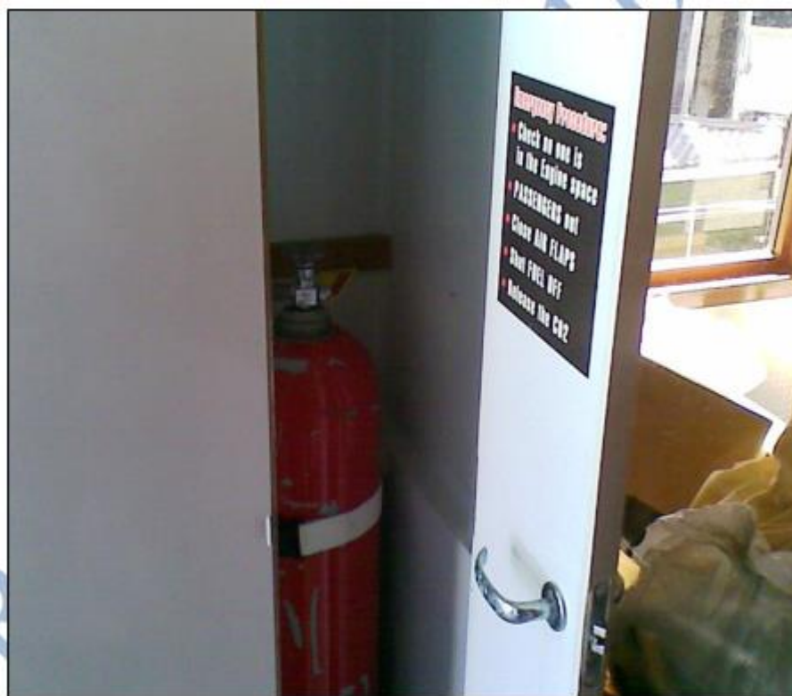
Figure 5 CO 2 locker showing the CO 2 bottle and its instructions for use
