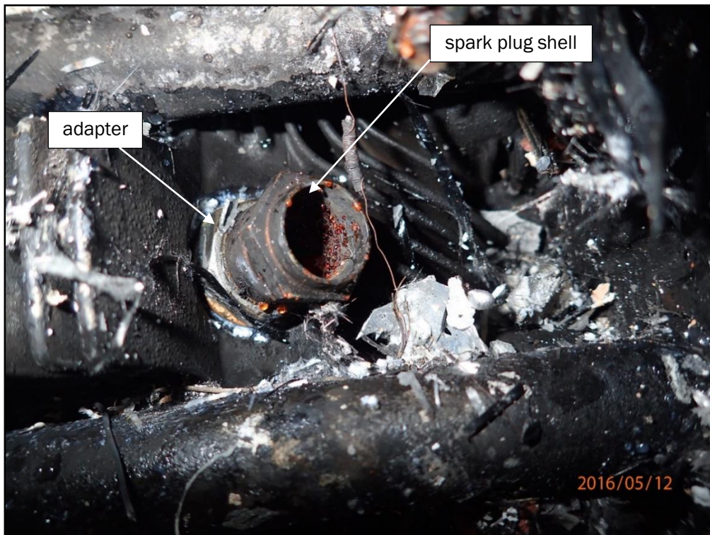
Figure 6 Failed number 4 cylinder upper spark plug shell
