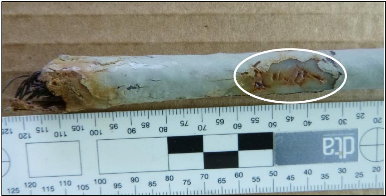
Figure 3. Penetrations of the outer sheathing 60 – 70 mm from failure
