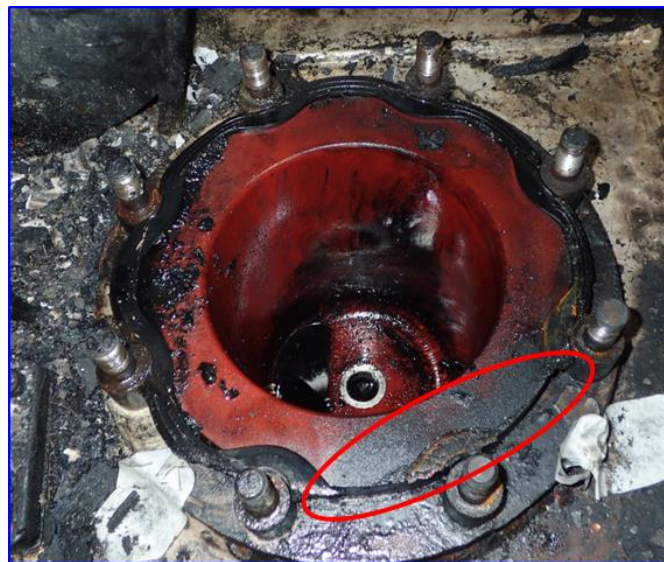
Figure 11 Damaged gasket between cable socket and oil-filled socket
