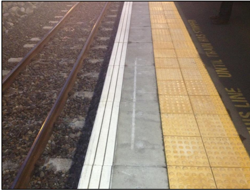
Figure 3 Witness mark from the mobility hoist on Waikanae Station platform
