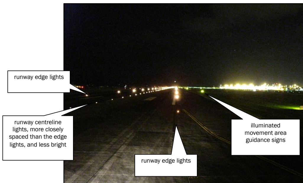
Figure 9 Runway 23 Left view while aligned with the edge lights (at cockpit height, 5.0 m above the surface)
