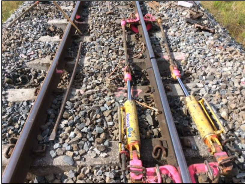
Figure 5 An example of rails being pulled together during a de-stressing operation
