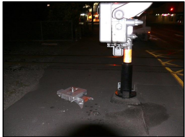
Figure 2 Damage to Moore Street level crossing barrier arms (photographs from KiwiRail)
