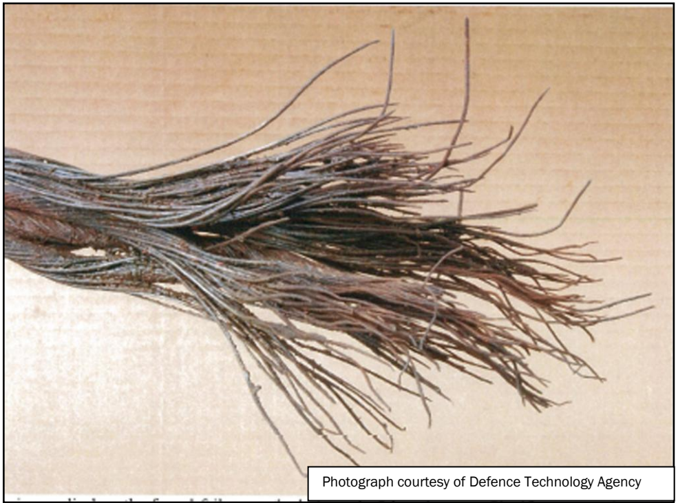
Figure 8 Photograph of the failure point of number 7 lifeboat forward wire fall
