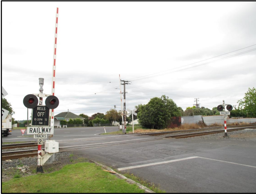
The Crown Road level crossing (located near Paerata)
