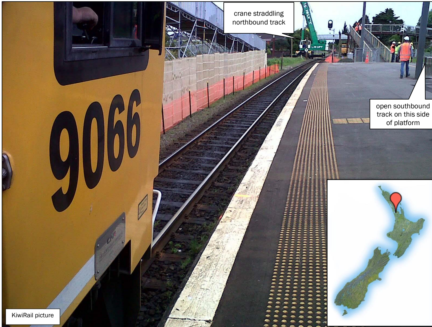
Train 228 stopped on the closed northbound track at Puhinui
