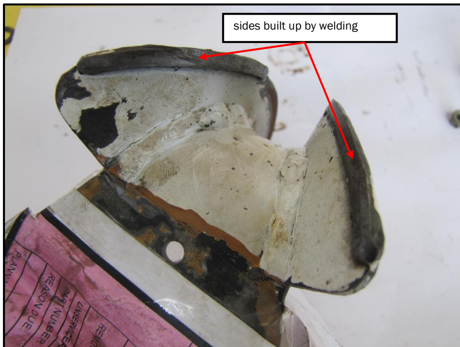
Figure 7 Alignment guide after removal, 11 April 2011, showing built-up sides
