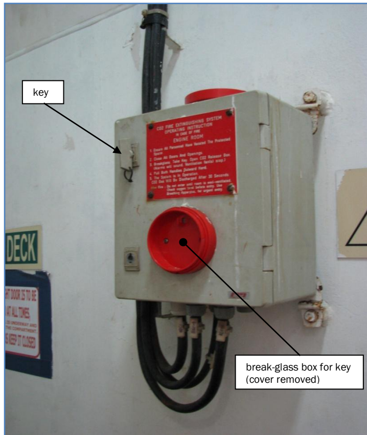
Figure 3 CO 2 system remote release box
