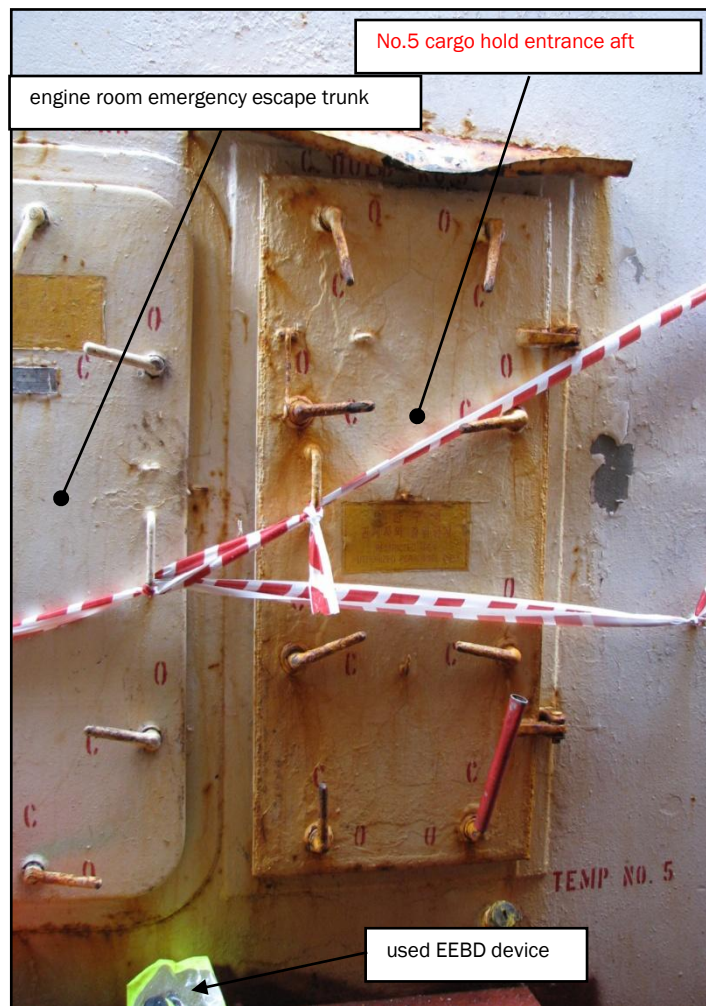
Figure 2 Entrance door to No.5 Cargo Hold aft
