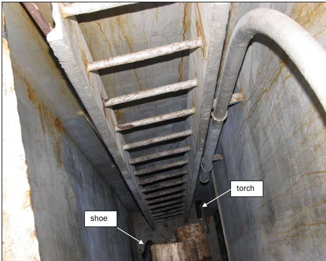
Figure 4 No.5 hold aft access showing shoe and torch unable to be recovered due to foul atmosphere
