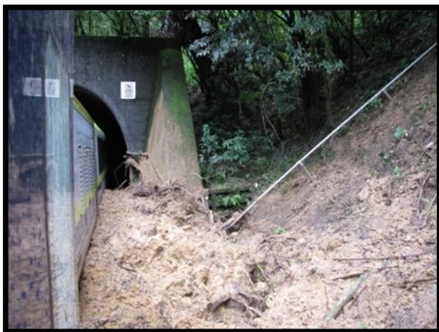
Figure 3 Portal 2, Left-hand side
