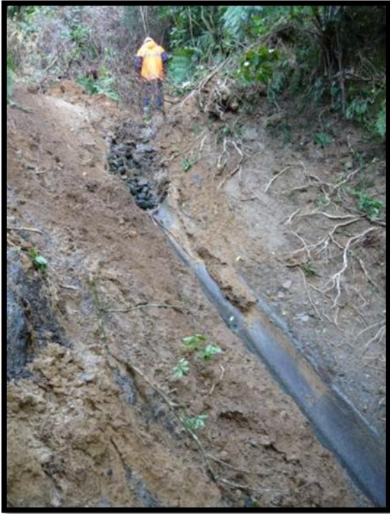
Figure 5 Formed drainage chute
