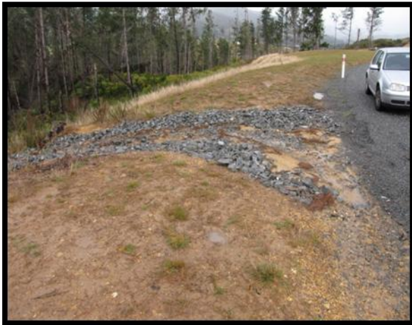
Figure 8 Drainage from ridge towards tunnel
