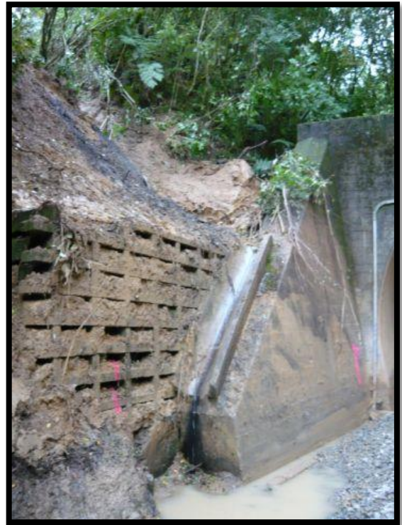
Figure 6 Portal 2, Drain to track
