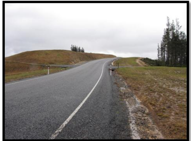
Figure 9 Cleared ridge above tunnel
