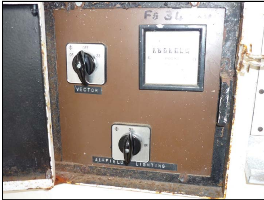
Figure 6 Aerodrome lighting remote control panel (New Plymouth District Council, 2009)
