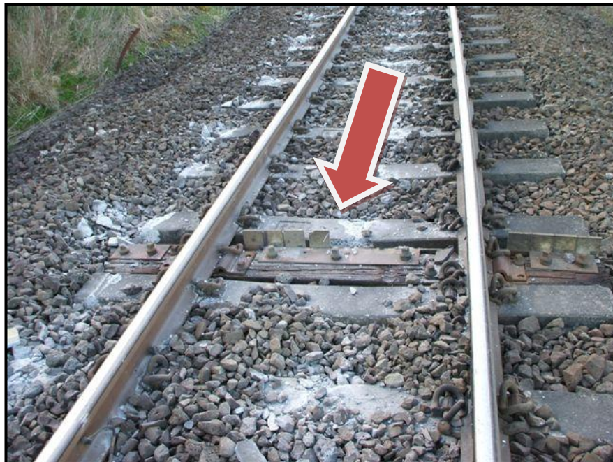
Figure 1 Damaged dragging equipment detector
