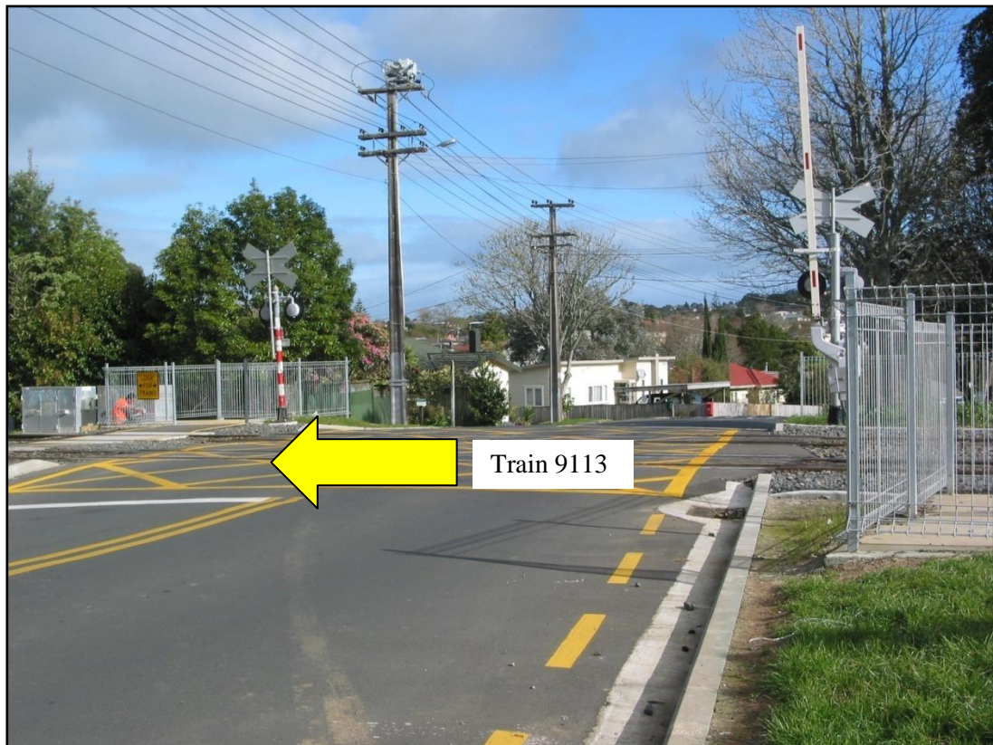
Figure 5 Fruitvale Road level crossing
