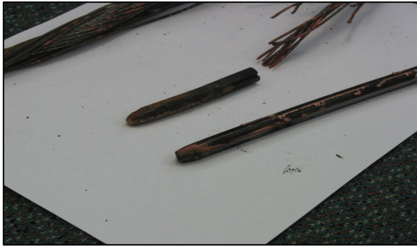
Figure 7 Parted overhead contact wire © Transport Accident Investigation Commission
