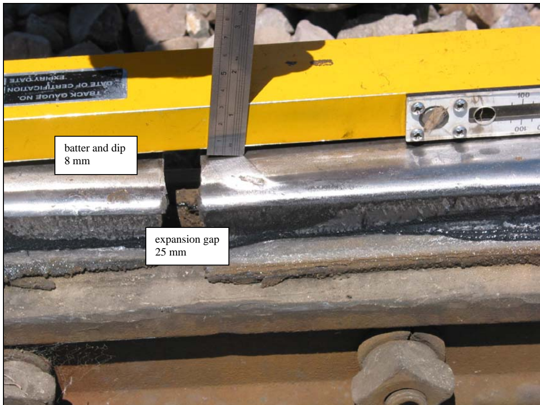
Figure 3 Termination joint at 309.642 km
