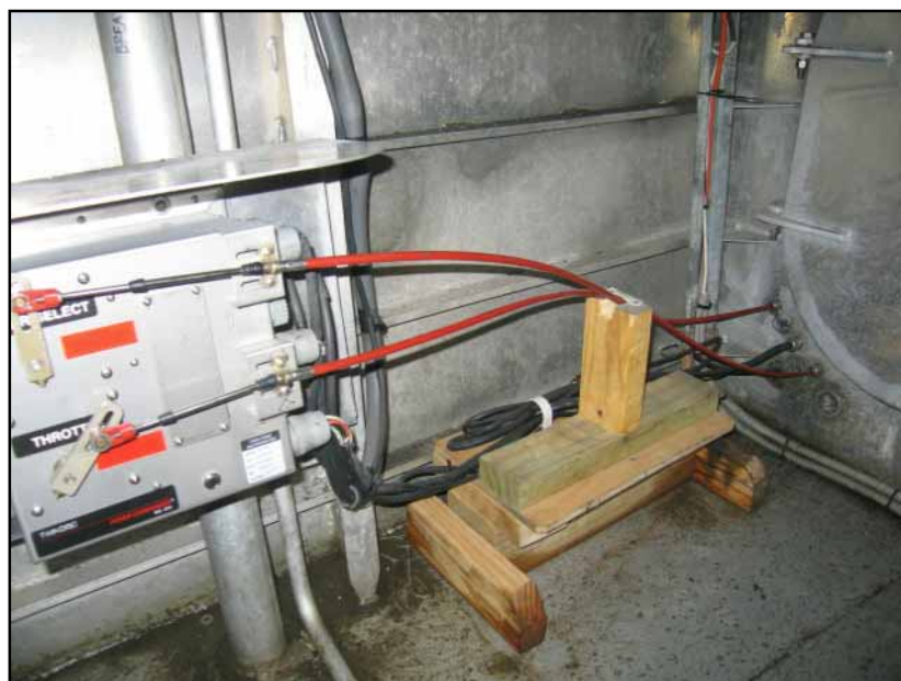
Figure 12 Control cable support as fitted after repairs
