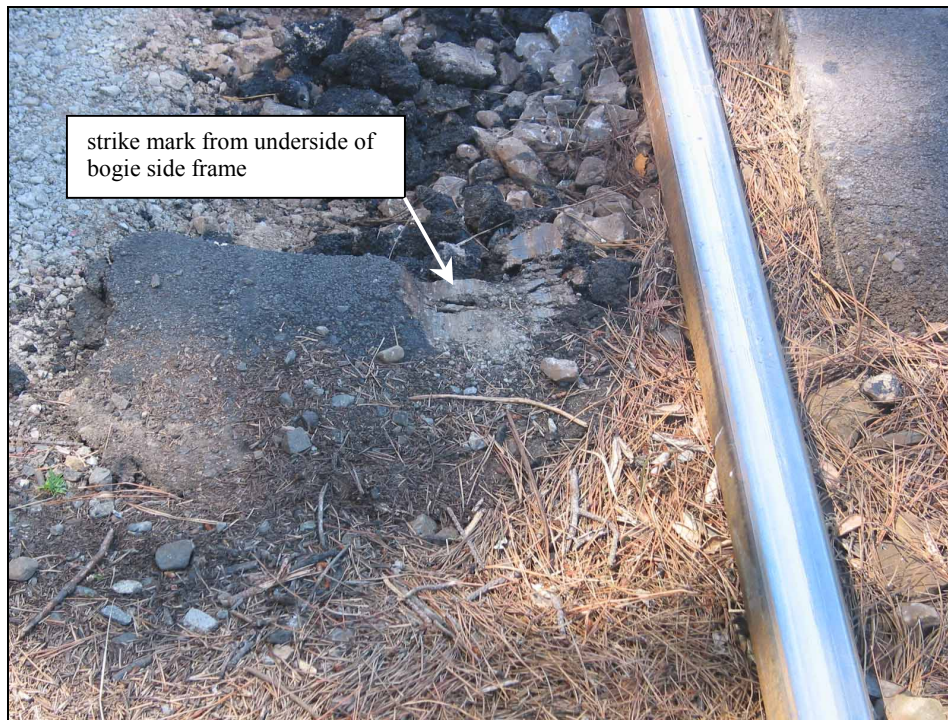
Figure 4 Pedestrian level crossing at Muri
