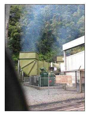
Figure 2 The extractor fan exhaust outlets at the western portal of the Otira Tunnel
