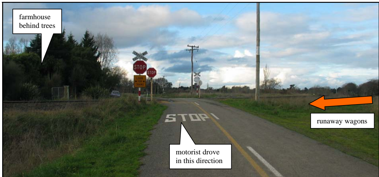
Figure 2 Hodders Road level crossing looking northwest
