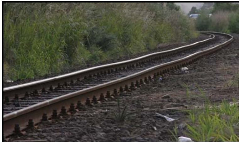
Figure 1 Track in the vicinity of the train parting location
