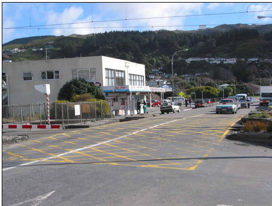
Figure 6 An example of yellow cross-hatching at a level crossing
