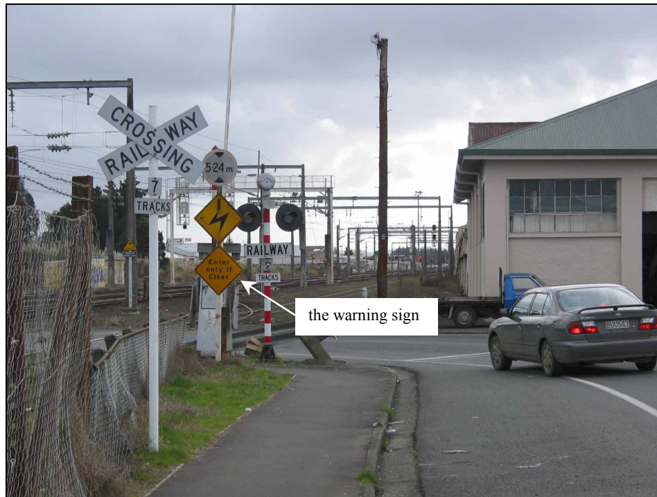
Figure 7 The overhead warning signs on the eastern side of the crossing
