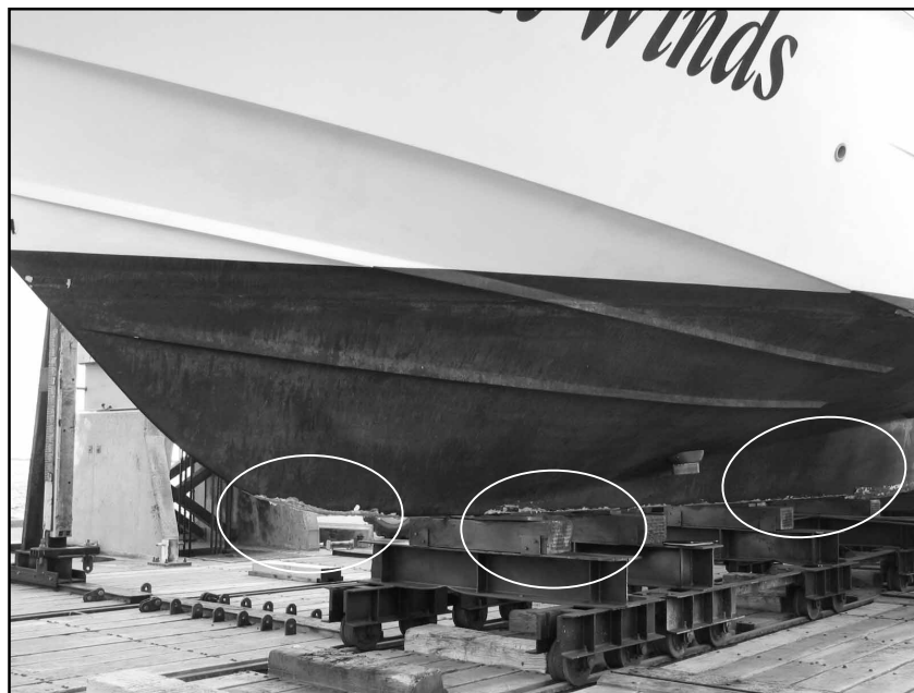
Figure 10 Areas of damage to the hull of the Southern Winds
