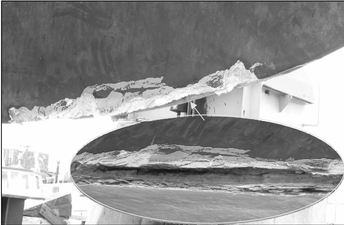
Figure 11 Damage to the bow of the Southern Winds
