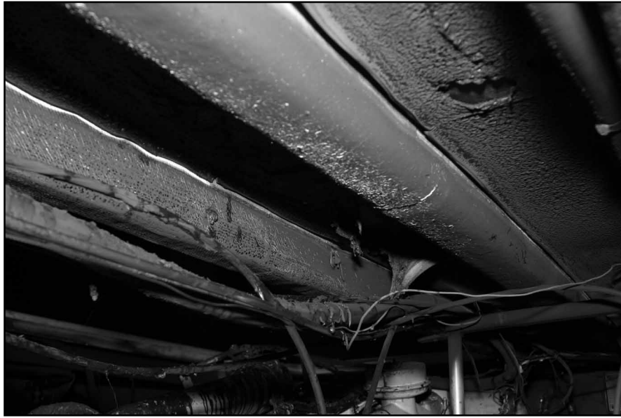
Figure 4 Deckhead above the port engine
