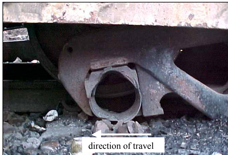
Figure 5 Bogie side frame of the derailed bogie
