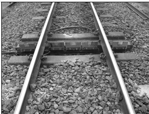
Figure 3 Combined heat/dragging equipment detection unit
