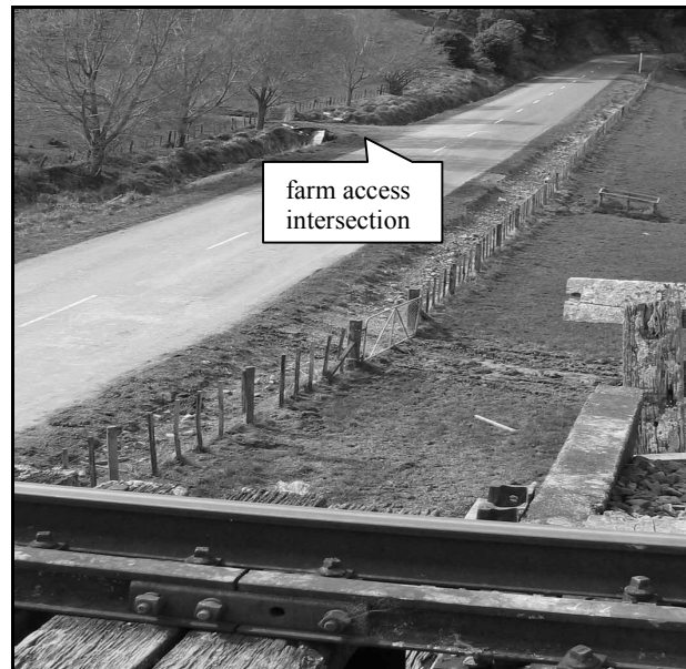
Figure 2 Opaki-Kaiparoro Road from top of bridge No.98 looking south to the farm access
