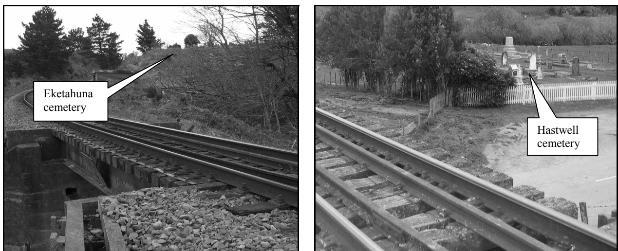
Figure 10 Bridge No.102 (left) and bridge No.98 (right) located next to cemeteries
