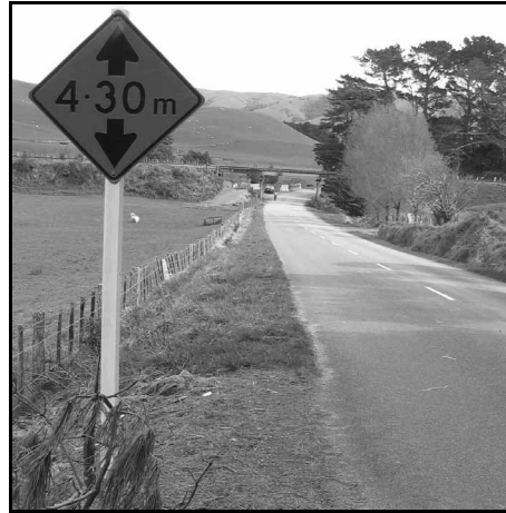
Figure 8 Looking north along Opaki-Kaiparoro Road towards bridge No.98
